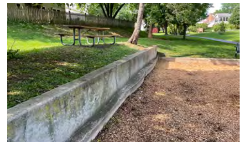
Playground retaining wall
