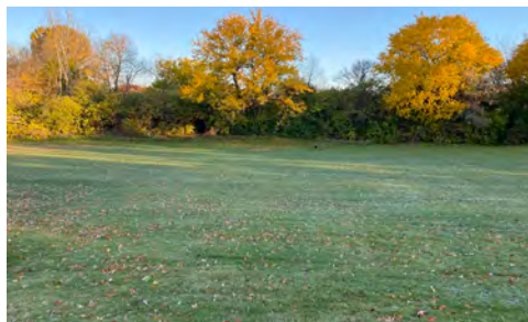
Detention basin and top of berm
