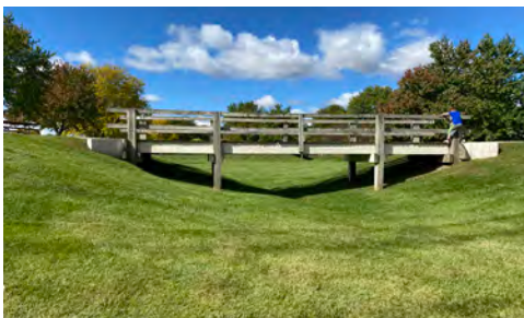
Detention basin / pedestrian bridge
