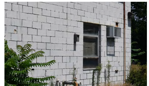
Tuck-pointing and windows
