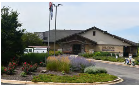
Front entry and drop-off
